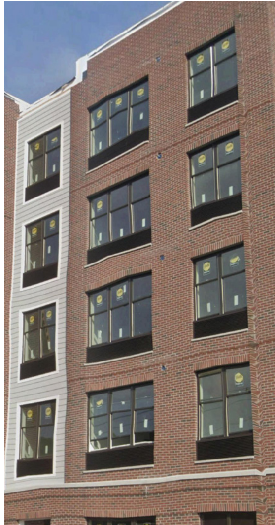
Through wall units integrated into window composition
